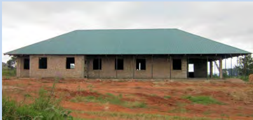
The clinic is now under roof...
