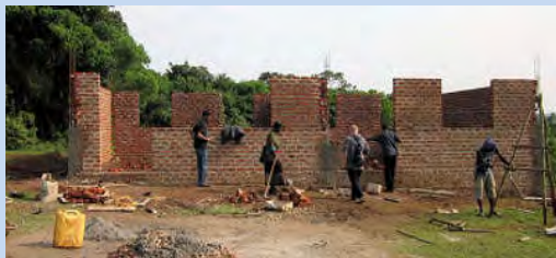
and the dormitory under construction.
